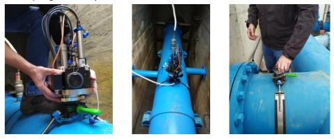
The user can easily remove the sensors for calibration without disturbing the installation or the water flow, completely safely for the users. *The system measures pH, Conductivity, Free Chlorine and it is expandable for measuring Turbidity, TOC, UV254, Colour, DOC*.
