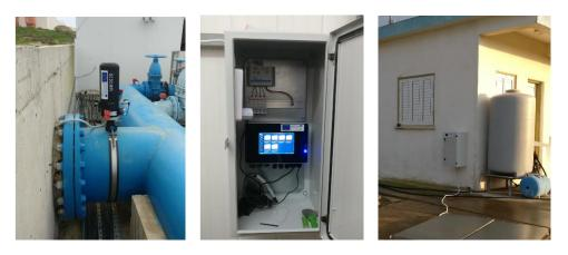
The systems measure and analyze the measurements every 5 minutes. The main advantage of these systems is the accurate measurements in perfect agreement to standardized lab reference, not just "trending", without interrupting the flow/pressure.
